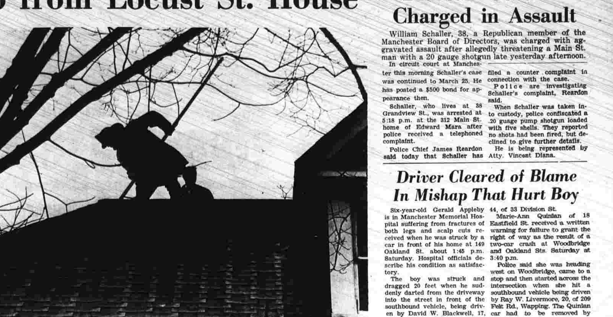
A fireman using a hook punches a hole in the roof of the 2 1/2-story house via an extension ladder from a fire truck parked many feet below.
